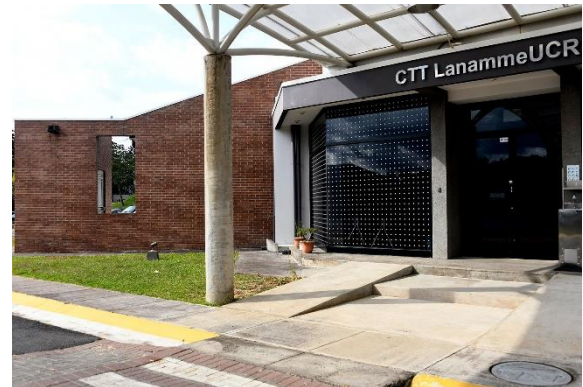
CCT del LANAMME, San Pedro
